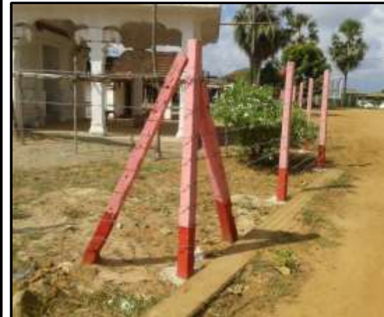
Renovation of Boundary Fence Sri Sinna velimalai Pillayar Temple
